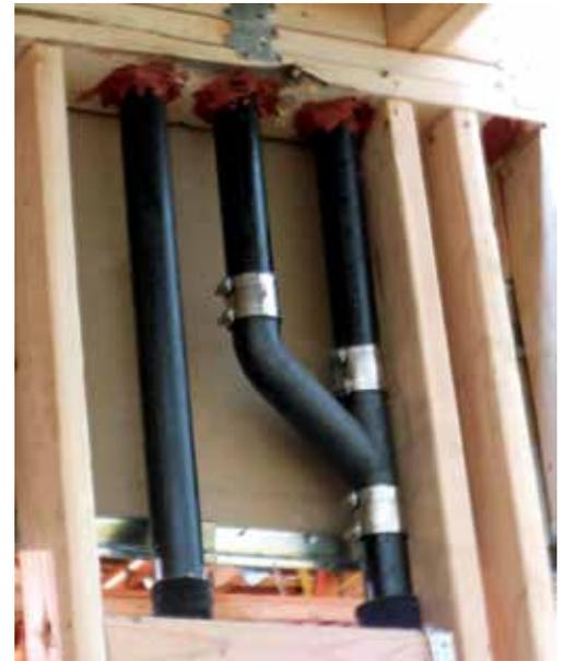
Plumbing joints with pipes nested in joint to allow for vertical movement of structure
