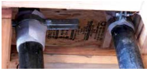
Plumbing sleeve connected to structure with foam wrap to allow vertical movement of structure
