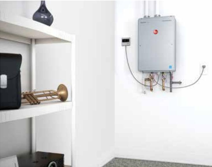
Indoor installation of a Rheem “Prestige” High Efficiency tankless unit serves a single apartment.
