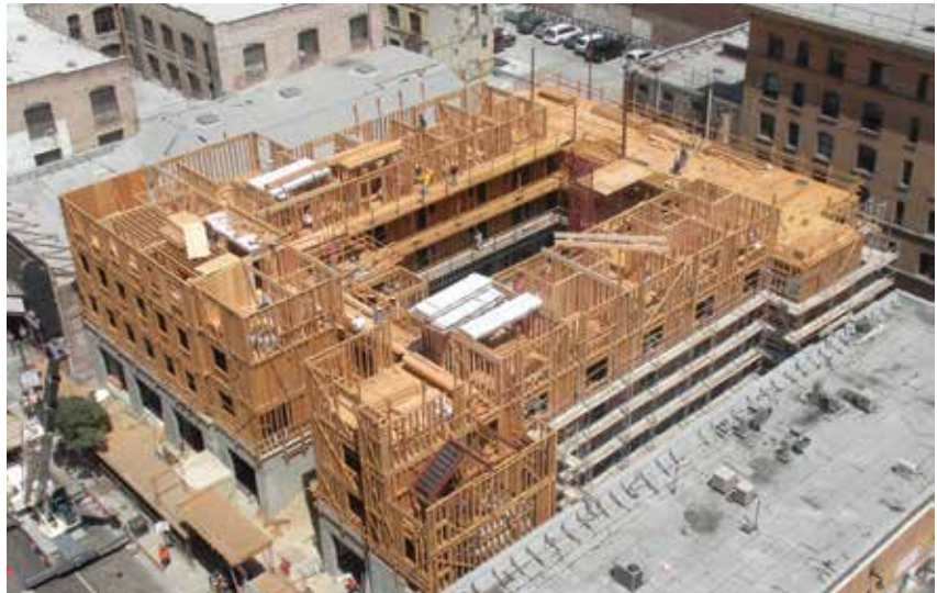
Photo: New Genesis Apartments, Killefer Flammang Architects, KC Kim, GB Construction
