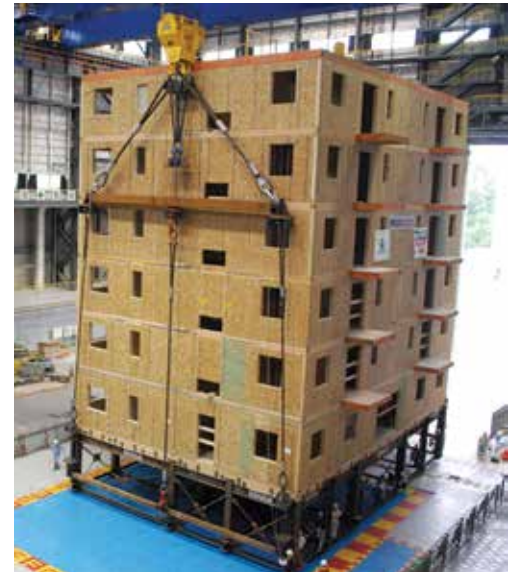
Subjected to three earthquakes on the world's largest shake table in Miki, Japan, this full-scale wood-frame apartment building performed excellently with little damage. Photo credit: John W. van de Lindt, Colorado State University
