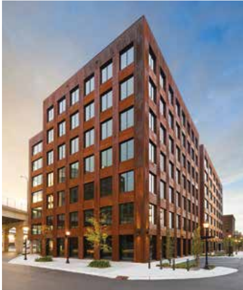
Approximately 3,600 cubic meters of wood are used in the T3 office building, in Minneapolis, which will sequester about 3,200 tons of carbon for the life of the building. The seven-story, 220,000-square-foot commercial building offers a mix of retail and office space.
