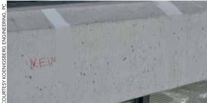
For River Plaza, in Chicago, Koenigsberg Engineering found that the more direct sunlight on the sloped portion of the repaired concrete exposed the repairs more glaringly than was the case on the vertical face.
