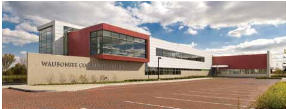
Holabird & Root employed a high-performance coating for the metal panels on Waubensee Community College in Plano, Ill. The panels (from Centria) are coated with a premium fluoropolymer (manufactured by Valspar) containing 70% polyvinylidene fluoride (PVDF) proprietary resins.
