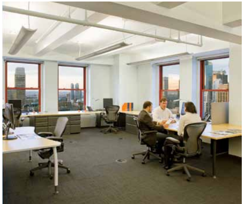
Arup engineers equipped Skanska's new headquarters in the Empire State Building with an electric light-dimming system that calibrates so effectively with daylighting levels that it is hard to perceive electric light output changes. Occupants are generally prevented from overriding the automated daylighting controls.
